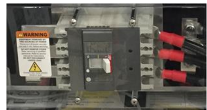
Figure 13: Battery breaker disconnect turned ON.
