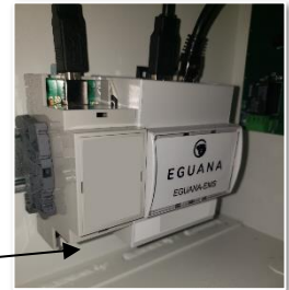
Figure 19: Meter communication connection.
