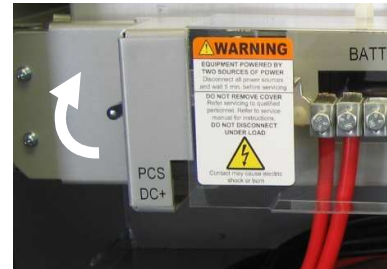
Figure 14: Battery breaker disconnect turn ON.
