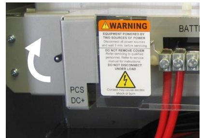
Figure 10: Battery breaker disconnect turn ON.
