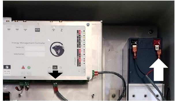
Figure 15: Connecting the AGM battery after permission to operate.
