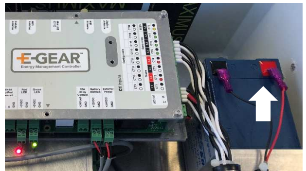
Figure 22: Connecting the AGM battery after permission to operate.
