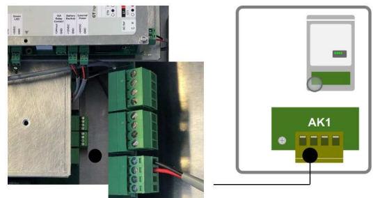
Figure 14: AK1 cable connection.
